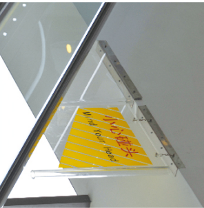
Perpendicular protection barrier (by client)
